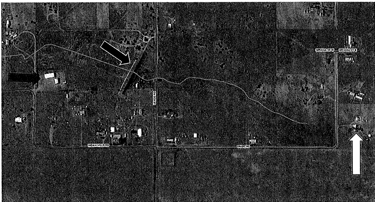
Figure 4. Some houses located downstream of the dam could potentially be flooded in the event of a severe storm. The black arrow shows the dam location. The white arrow shows one of several houses potentially at risk in the event of a severe storm.
